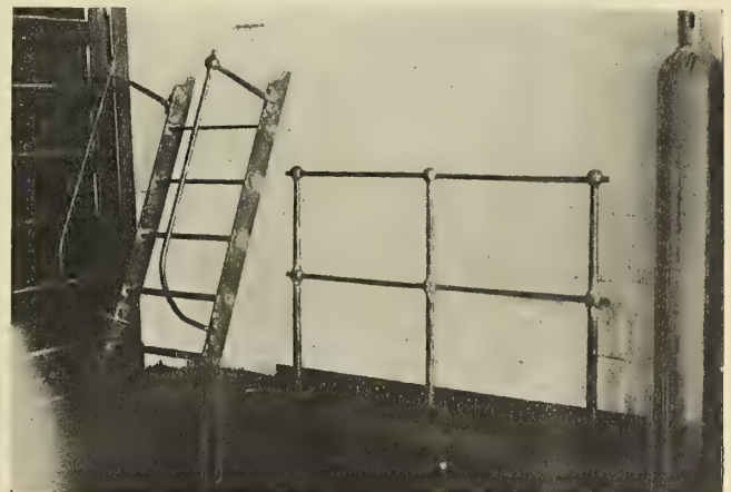
Fig. 2.—Left to Right: Ship's Ladder of Welded Construction by Oxy-Acetylene Process; Oxwelded Deck Rail, Welded to Deck Plating; Linde Oxygen Cylinder
